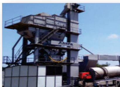
ASPHALT BATCH MIX PLANT
