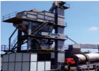
ASPHALT BATCH MIX PLANT
